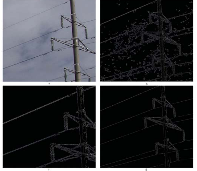
Fig. 3. Original image (a), Image after Canny filtering(b), Hough Transformed image (c) and Filtered image (d)
